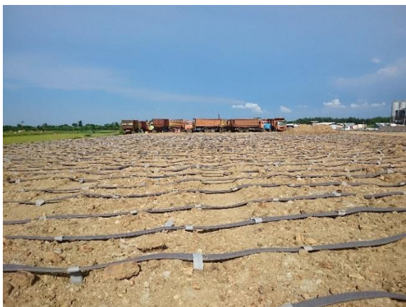
Figure 3. Installation of PVD and PHD
