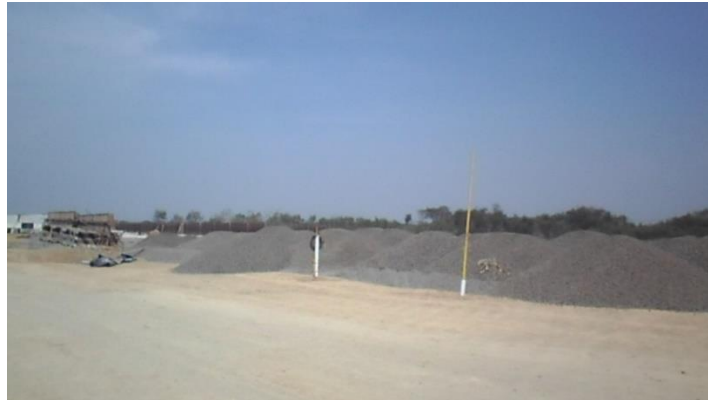
Figure 5. Installing the preload
