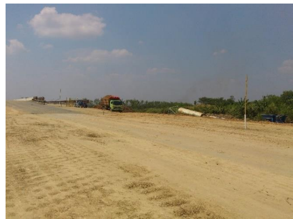
Figure 4. Installation of settlement plate instrument
