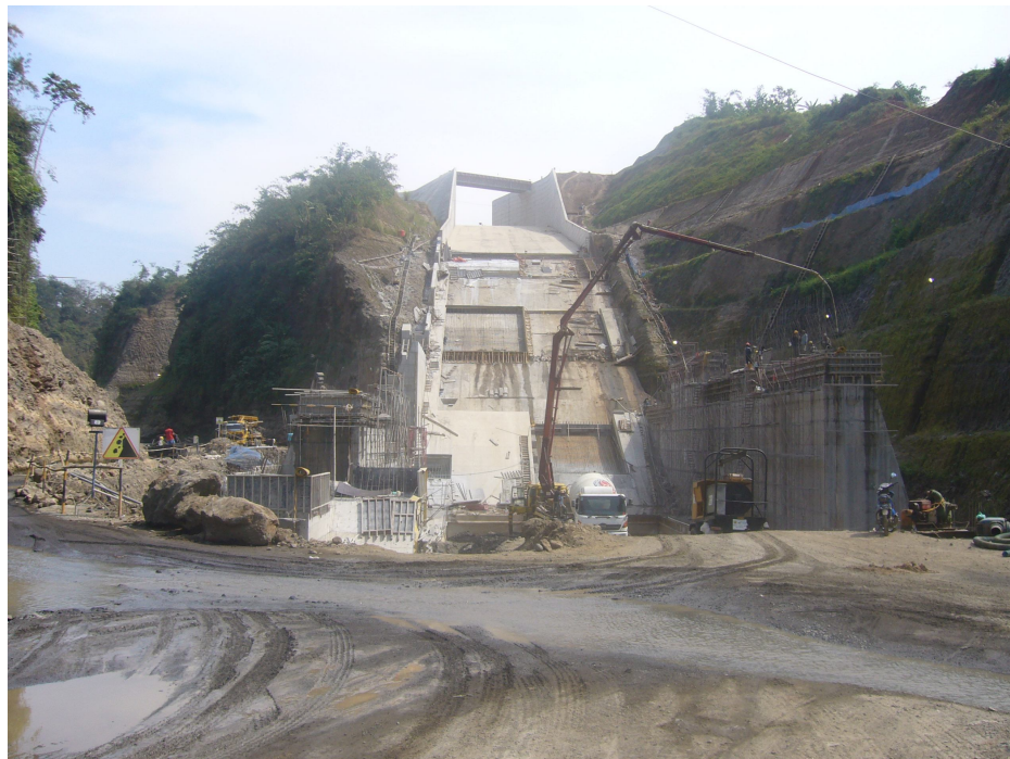
Figure 5 Spillway structure seen from the downstream
