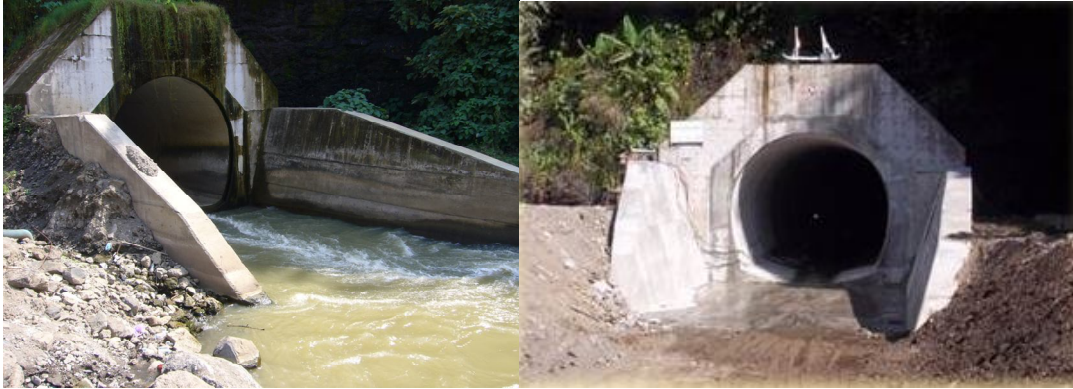
Figure 4 Intake and Outlet of the diversion tunnel
