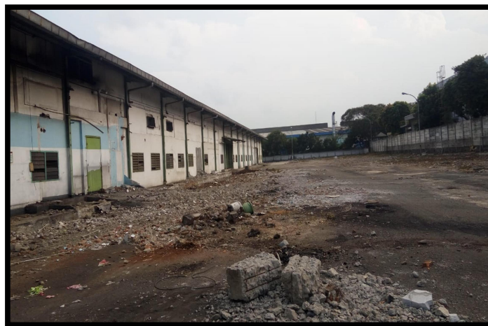
Gambar 2. Bangunan incondition pabrik A – 06 tampak samping Sumber: Peneliti, 2019
