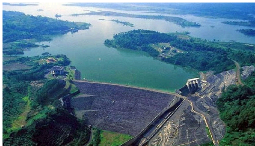
Figure 5. Saguling Dam in Bandung District, West Java.
